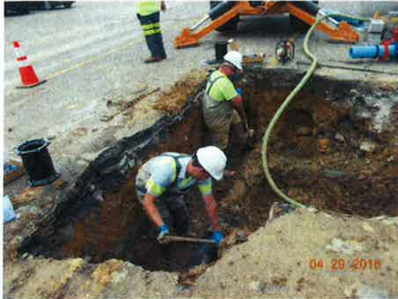
Hydrant Replacement & Leak Repair
