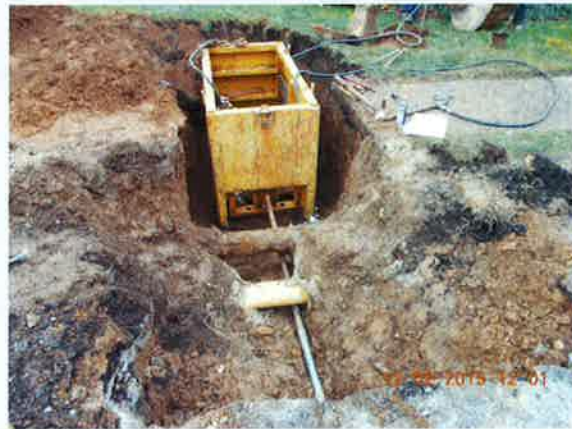
Service Install with Road Bore
