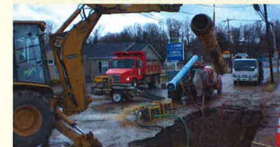
Main Line Repair
