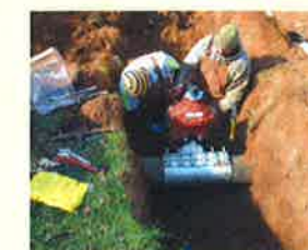
Valve Installation
