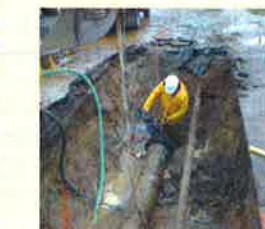
Main Line Repair
