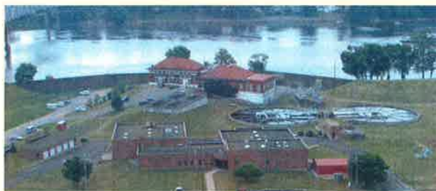
Water Treatment Facility
